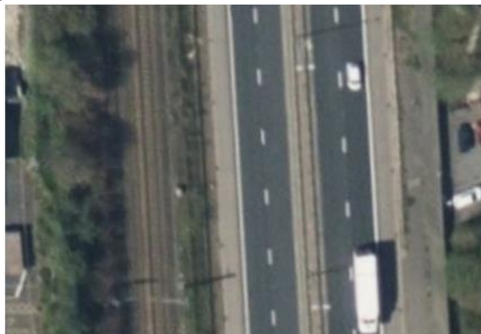
View of Liverpool & Manchester Railway in close proximity to M602 Distance from running rail to motorway hard shoulder is circa 7m.
