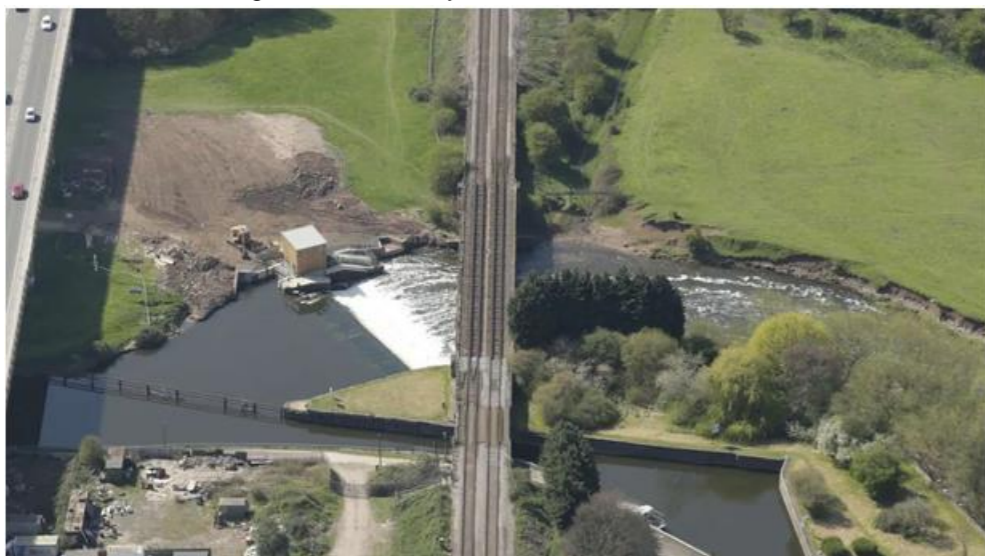
River Devon Trent showing the weir and Hydro-Electric Power station
